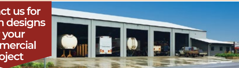
LARGE MACHINERY SHED
